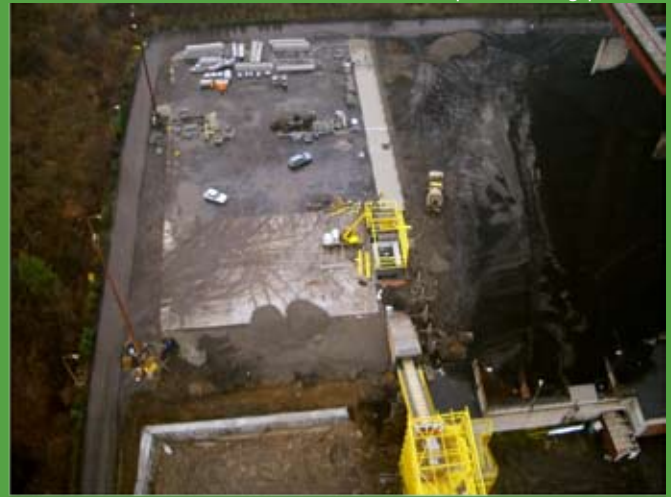
distribution of dump – building process
