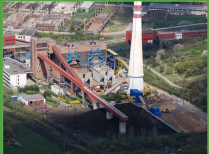
heating plant after reconstruction
