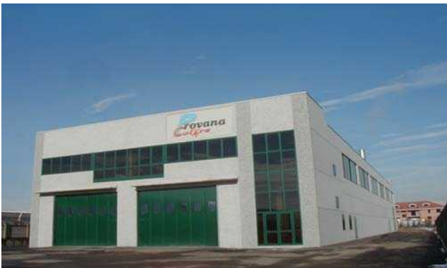
Photo: District Heating plant
