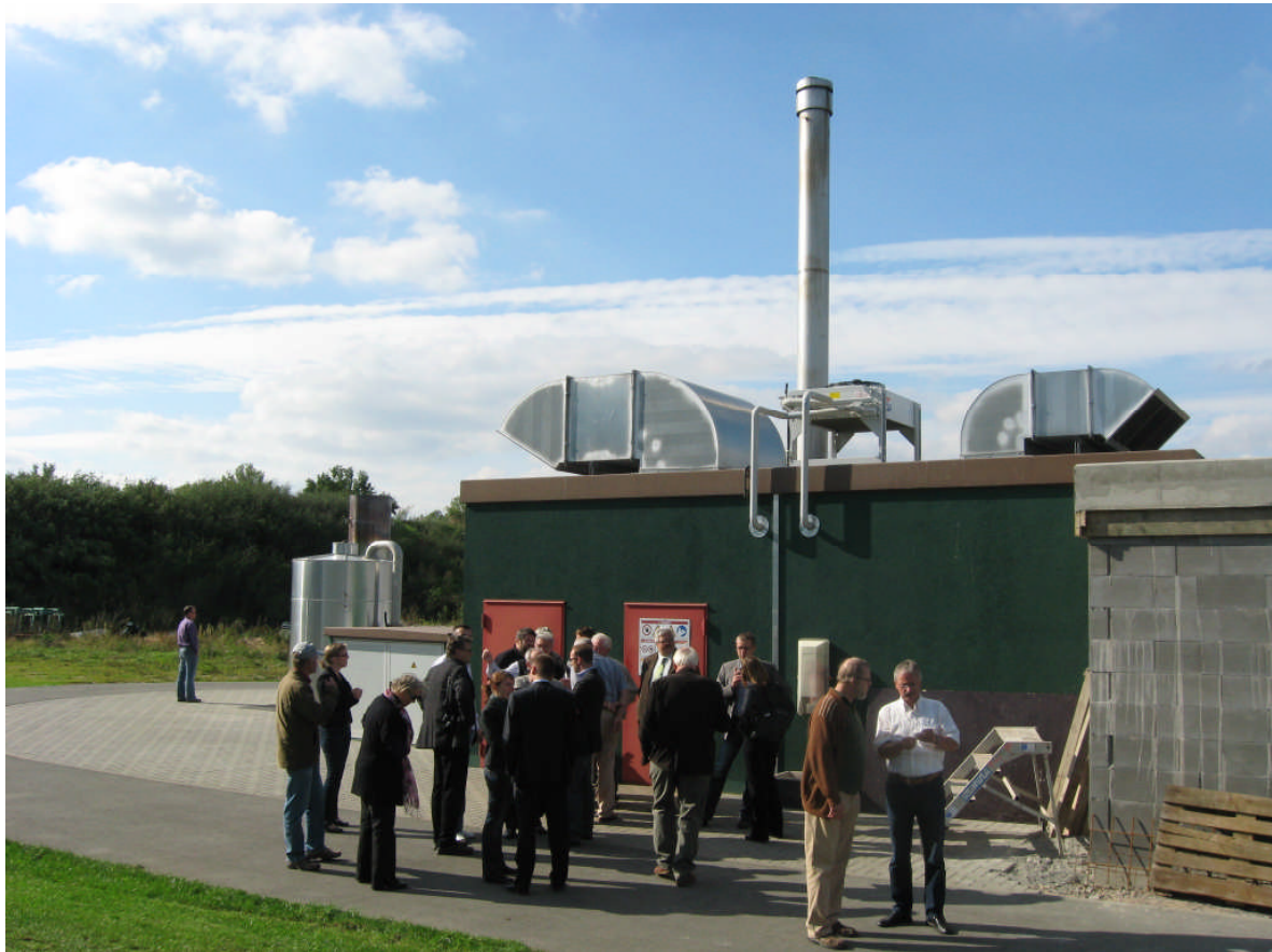
Picture 3 The cogeneration plant in Tangeln
